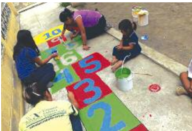
GUATEMALA. Renovierung eines Kinderheims GUATEMALA. Repairs to a Children's Home
